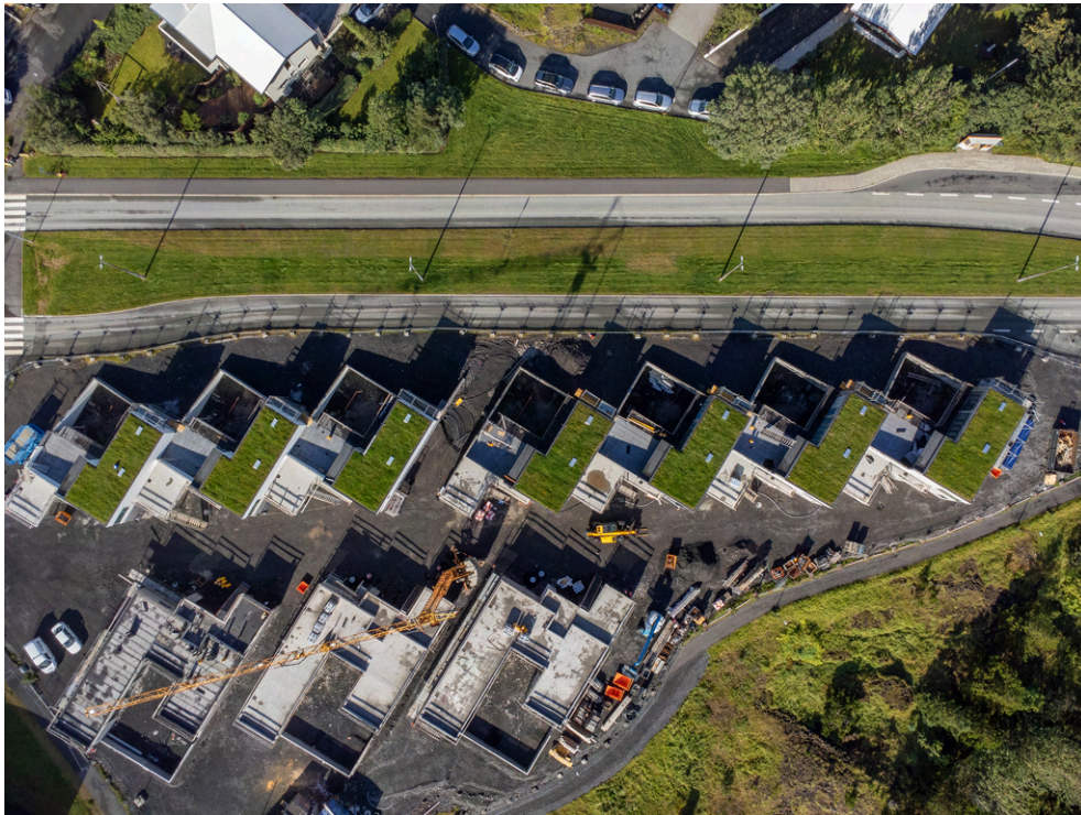
Photo: Róbert Magnússon, Hjallabraut 49, Hfj. Construction site, Iceland, summer 2024
